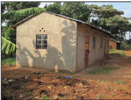
The new cooking hut at Vigena Primary School, complete with an energy efficient stove.
